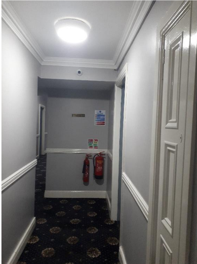
Corridor/CCTV/ Fire Extinguishers
