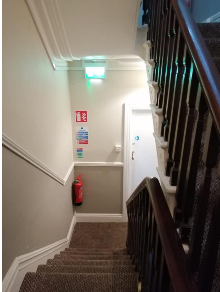
Stairs, Fire notices, fire door
