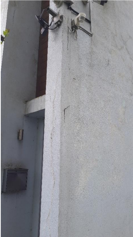
Exterior of Building
