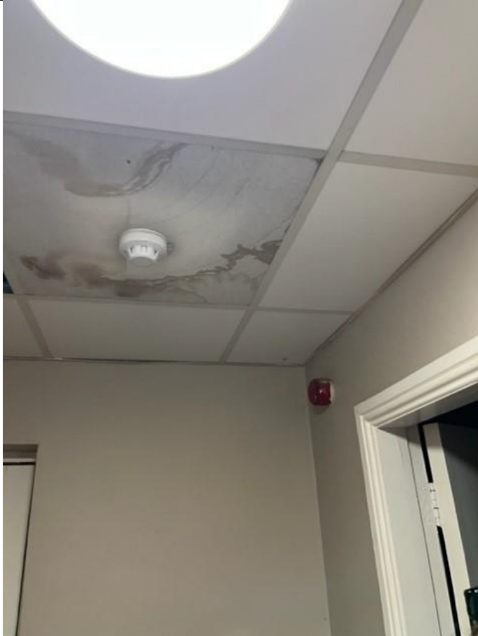
Ceiling Leakage
